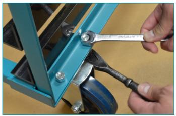
Figure 8. Attaching non-locking rear casters to bottom cross members and upright.
